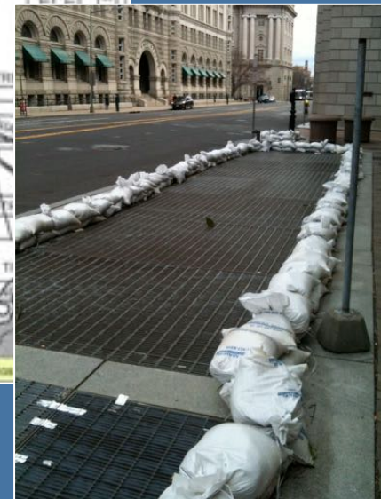
WMATA stormwater barriers
