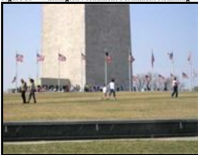
Figure 26 – Washington Monument Permanent Retaining Walls
