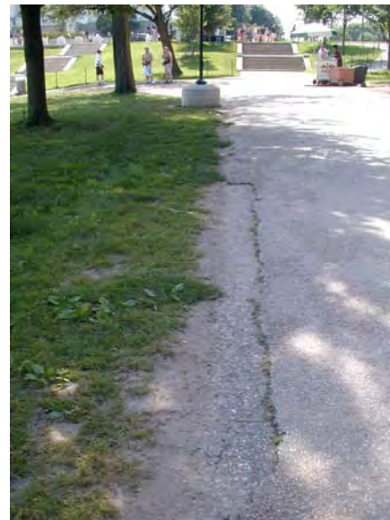
Figure 3.2 – Example of uneven pavement along the north elm walk
